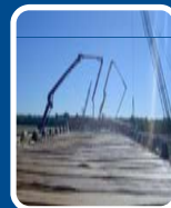
CO 2 concrete curing
